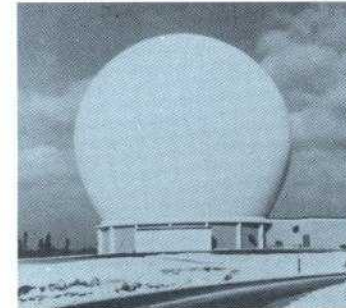
Mill Village, Canada
