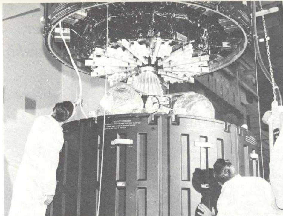
Engineers at Hughes Jet Propulsion Laboratory in Pasadena, Calif., check the fit of the solar cell casing on the INTELSAT IV satellite now in production. Launching of the Series IV satellite is scheduled by INTELSAT for mid-1971.
