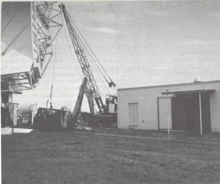
The hydramech, a large variable volume pump and reservoir, is moved from the transportable station antenna pedestal to the recently completed building.
