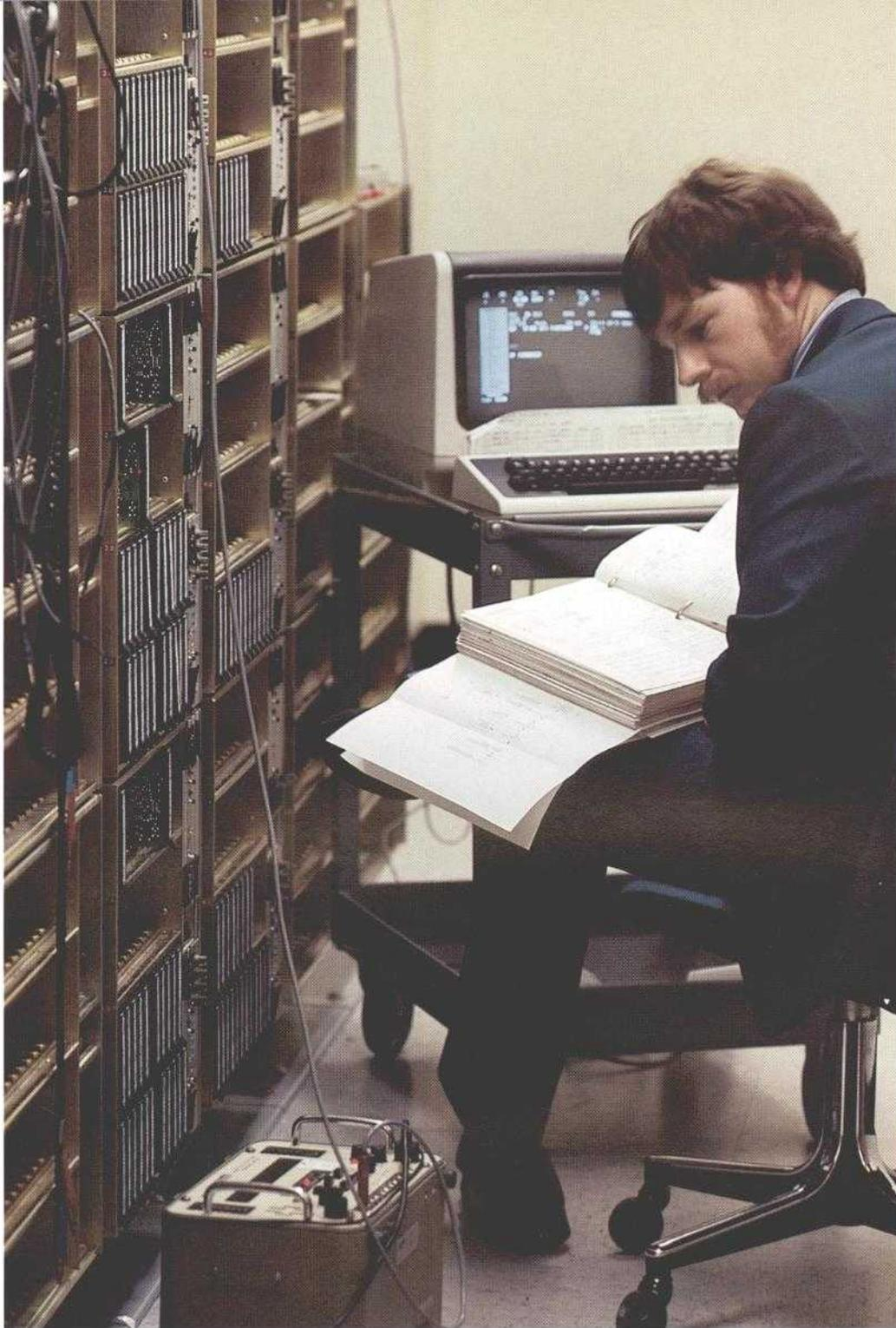
**Left,** SBS field engineer working on channel banks terminating equipment at the MS-I Network Access Center in downtown Atlanta. **Below,** MS-I is for those telephone users with a medium to high volume long distance requirement.
